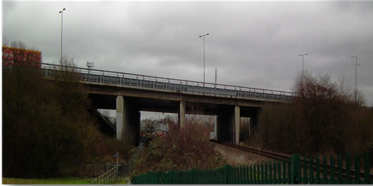
Figure 3233 View of Windsor Branch Railway Bridge from the South
