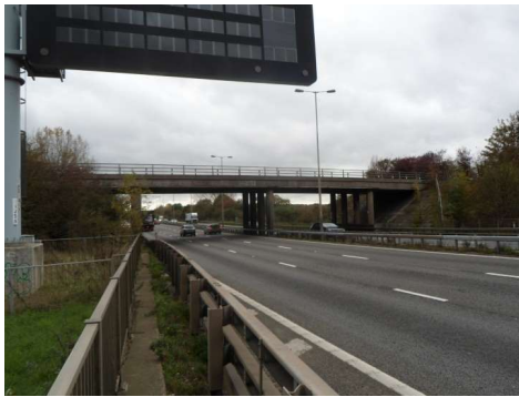
Figure 2 View of the existing Monkey Island Bridge
