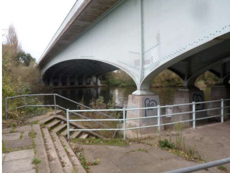
Figure 253 View of Thames Bray underbridge from south-east embankment
