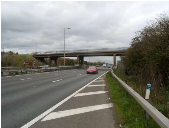
Figure 3030 3030 View of the existing Wood Lane bridge
