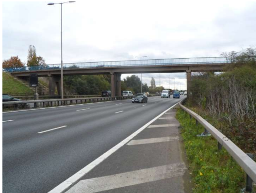
Figure 3435 View of the existing Recreation Ground bridge
