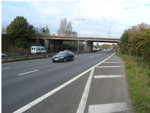
Figure 6 View of the existing Datchet Road bridge
