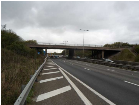
Figure 1 View of the existing Ascot Road Bridge
