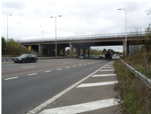
Figure 2828 View of the existing Huntercombe Spur bridge
