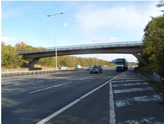
Figure 7 View of the existing Old Slade Lane bridge
