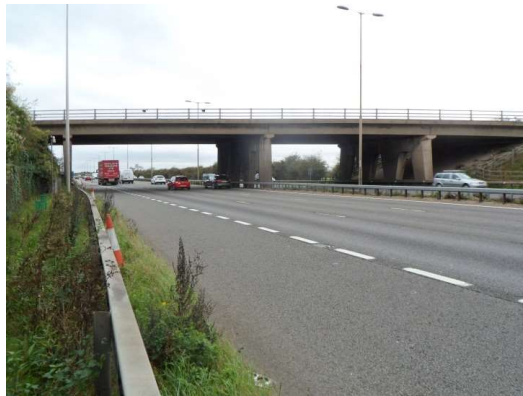
Figure 5 View of Existing Lake End Road bridge
