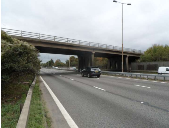
Figure 4 View of the existing Marsh Lane bridge
