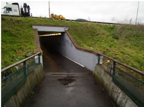
Figure 38 Langley Interchange subway
