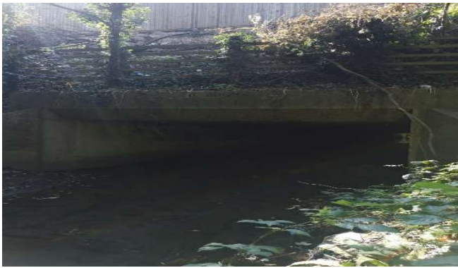
Figure 32 View of Railway culvert from the North
