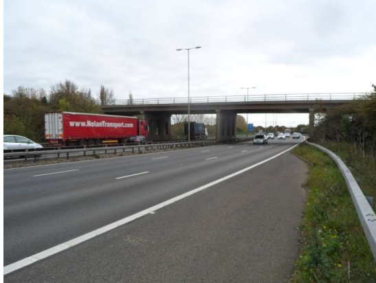
Figure 3536 View of the existing Riding Court bridge
