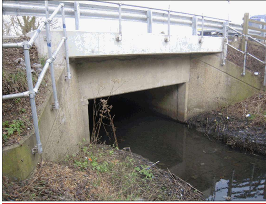
Figure 3431 View of the southern of Chalvey culvert
