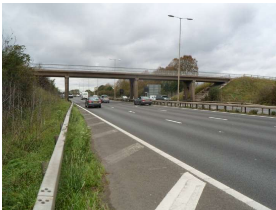
Figure 2929 View of the existing Oldway Lane bridge
